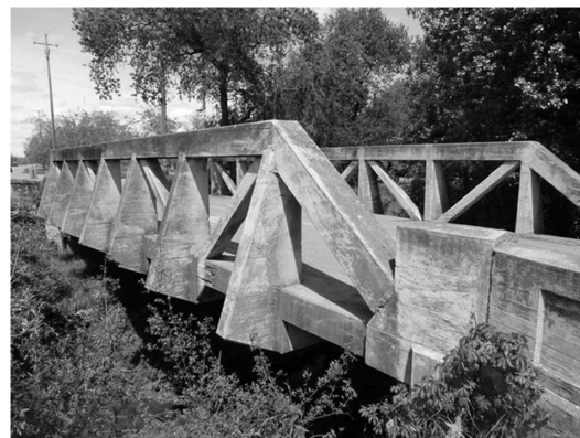
Concrete Truss – Kilburn Rd. Bridge, Calif.
