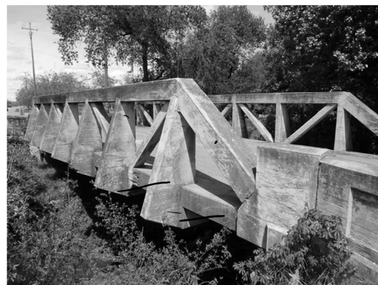
Concrete Truss – Kilburn Rd. Bridge, Calif.
