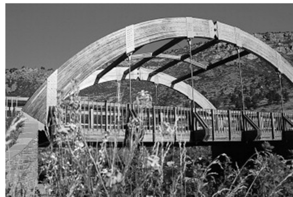
Hinged Glulam Timbers
