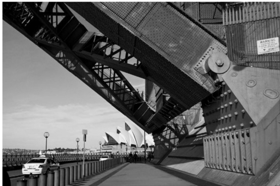
Sydney Harbour Bridge
