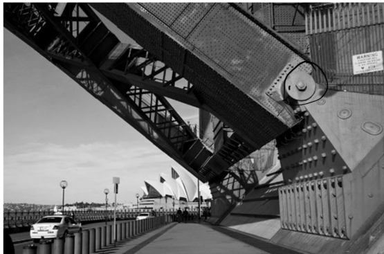
Sydney Harbour Bridge
