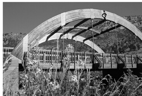
Hinged Glulam Timbers
