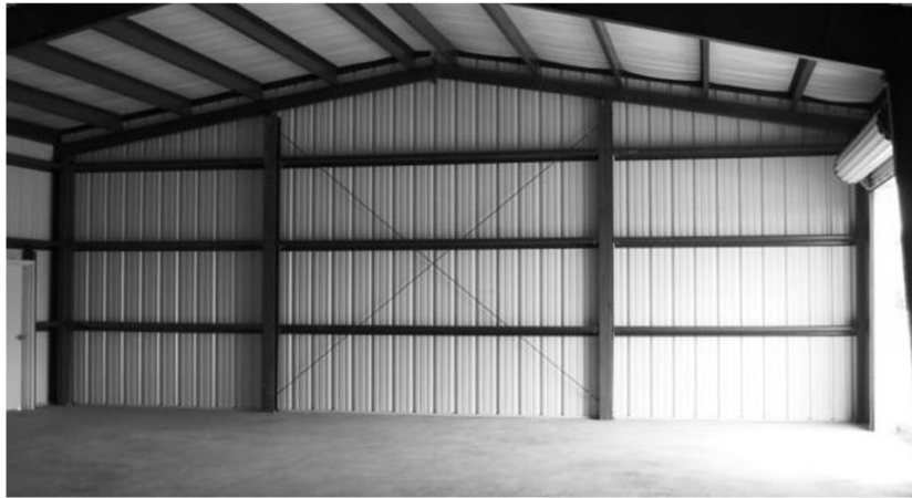
Diagonal Tension Counters (X-Bracing) (Buck Steel Buildings)
