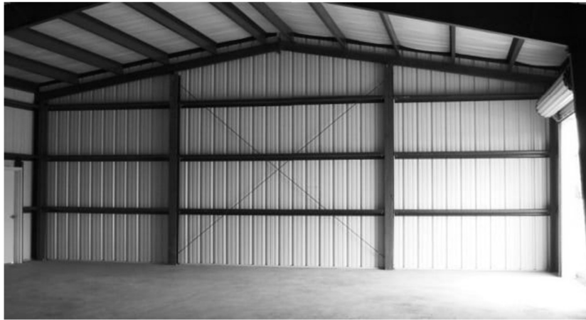
Diagonal Tension Counters (X-Bracing) (Buck Steel Buildings)
