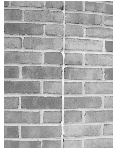
Expansion joint in wall
