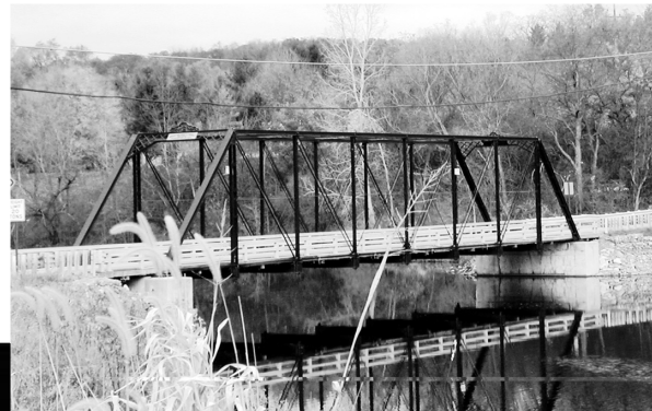
Foster Bridge, 1889 Ann Arbor, Michigan
