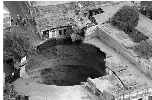
Subsidence (Pierces, Guatemala)
