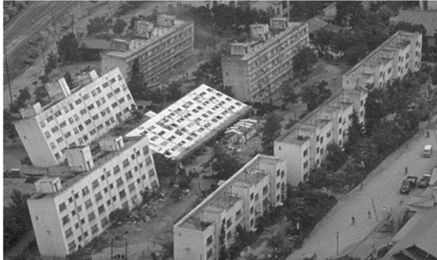
Liquefaction (Niigata, Japan 1964)
