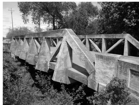
Concrete Truss – Kilburn Rd. Bridge, Calif.
