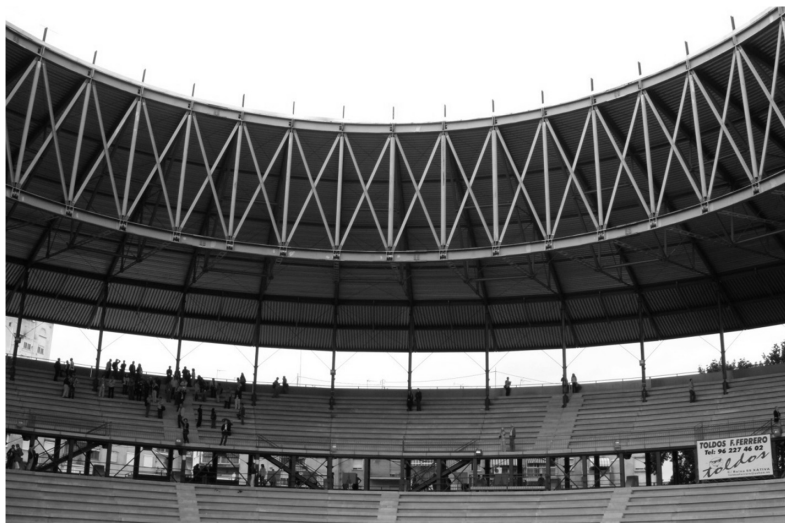
Bullring Covering, Xàtiva, Spain Kawaguchi and Engineers, 2007
