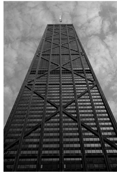
John Hancock Tower - 1968 875 North Michigan Avenue, Chicago Fazlur Kahn, SOM
