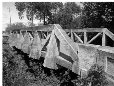
Concrete Truss – Kilburn Rd. Bridge, Calif.
