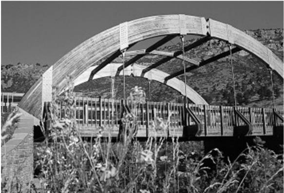
Hinged Glulam Timbers
