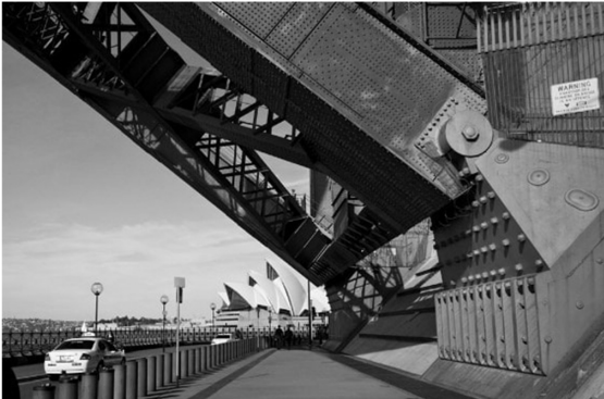
Sydney Harbour Bridge
