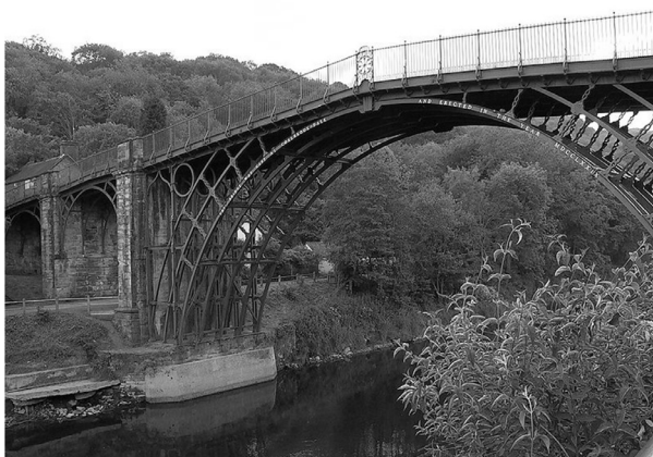
The Iron Bridge Telford England
