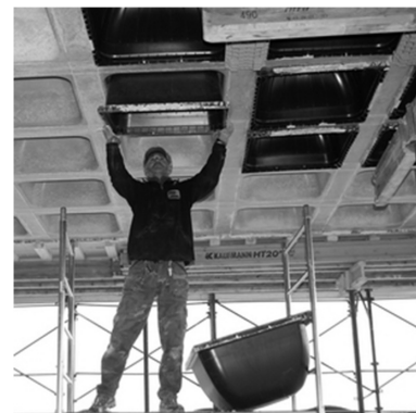
two-way waffle slab
