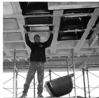
two-way waffle slab
