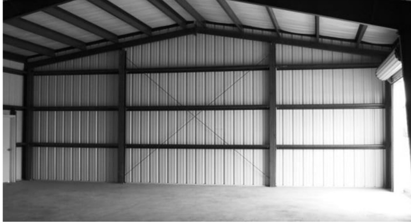
Diagonal Tension Counters (X-Bracing) (Buck Steel Buildings)
