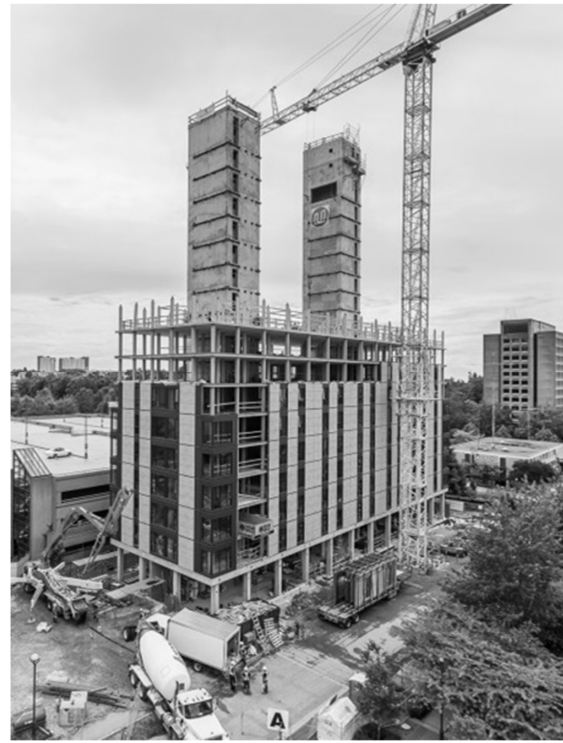
Brock Commons Tallwood House University of British Columbia, Vancouver, Canada
