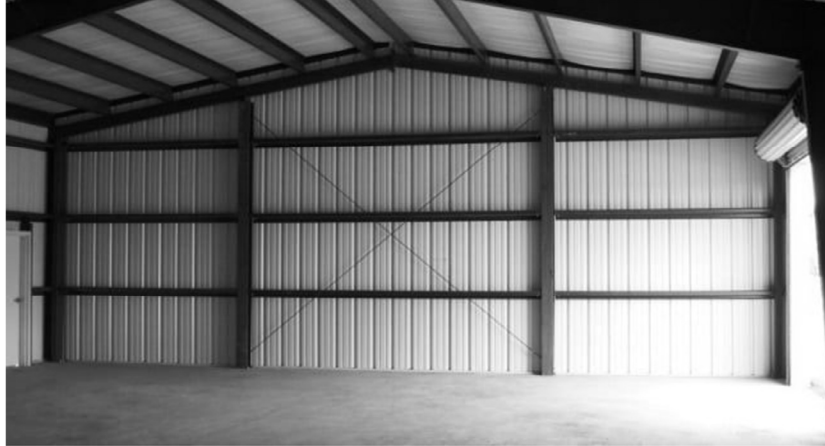
Diagonal Tension Counters (X-Bracing) (Buck Steel Buildings)
