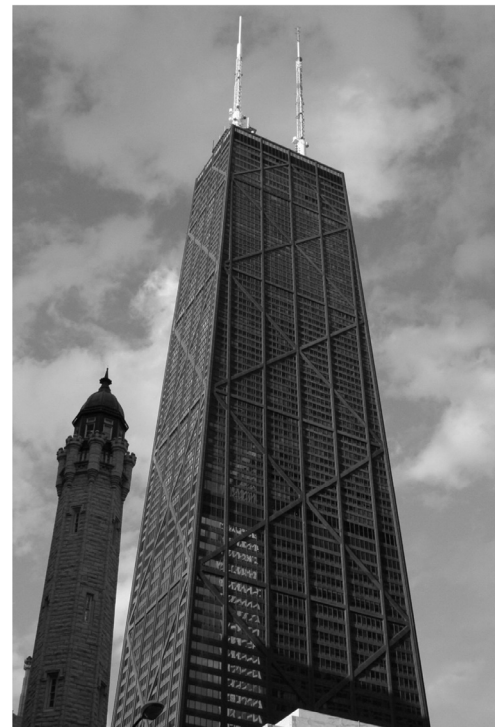
John Hancock Tower, Chicago SOM, 1968 Engineer: Fazlur Khan
