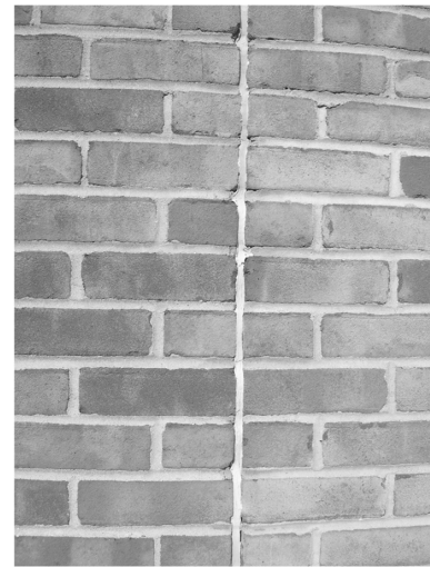
Expansion joint in wall
