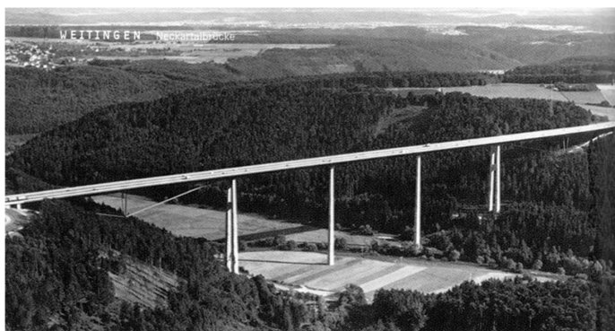
Cable supported span of 866 ft Jack height of 118 ft Cable length 895 ft
