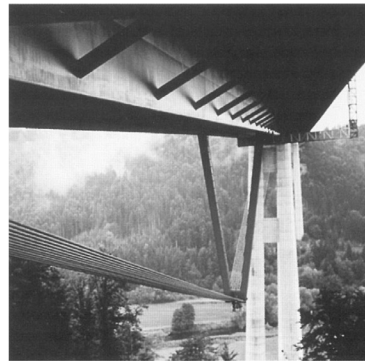
Cable supported span of 866 ft Jack height of 118 ft Cable length 895 ft
