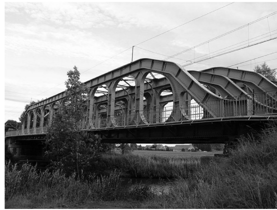
Vierendeel bridge at Grammene, Belgium Photo by Karel Roose
