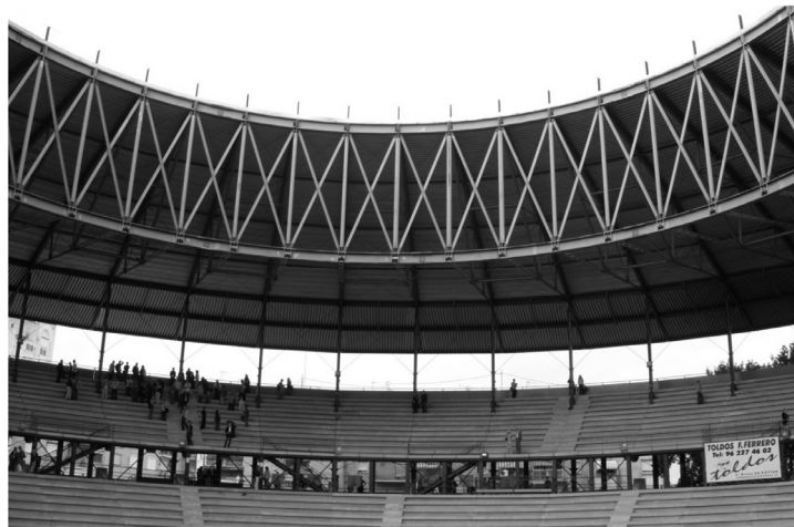
Bullring Covering, Xàtiva, Spain Kawaguchi and Engineers, 2007
