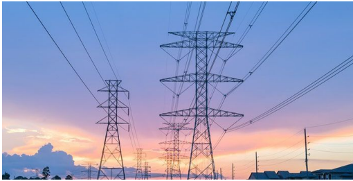
Transmission Cable Lines
