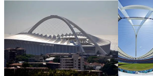
Arch tower cable supported roof, Moses Mabhida Stadium, South Africa
