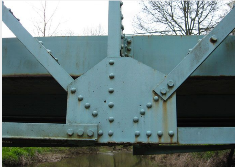
Bridge Gusset Plate
