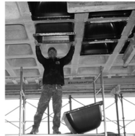
two-way waffle slab
