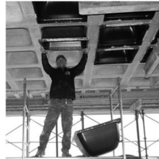
two-way waffle slab
