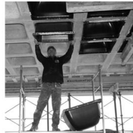
two-way waffle slab
